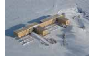
New South Pole Station
