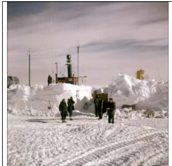
Control Tower at Little America V taken in 1957
