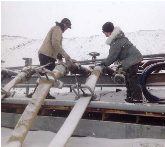
Photo by Sarah Burford Crews on the McMurdo Station ice-pier attach hoses and prepare to discharge fuel from the MSC chartered ship MT Maersk Peary.
