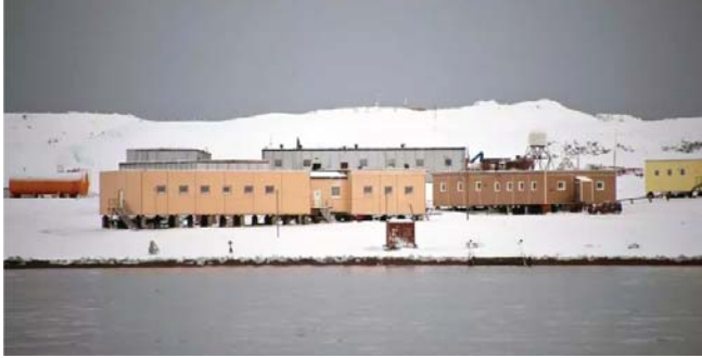
Photo by Vanderlei Almeida Partial view of Bellingshausen Station
