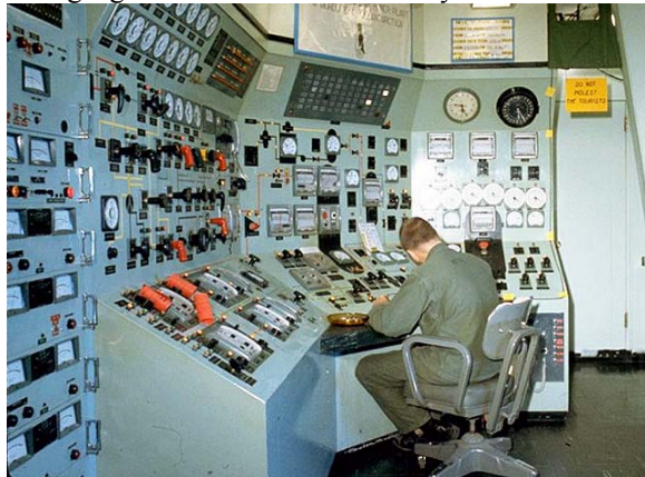
PM-3A Control Room
