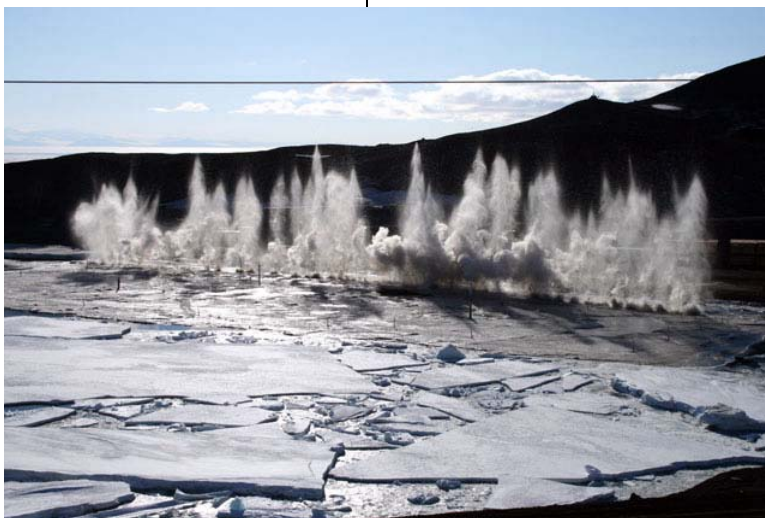
Photo Credit: Carlie Reum Explosives dislodge the ice pier from Winter Quarters Bay.
