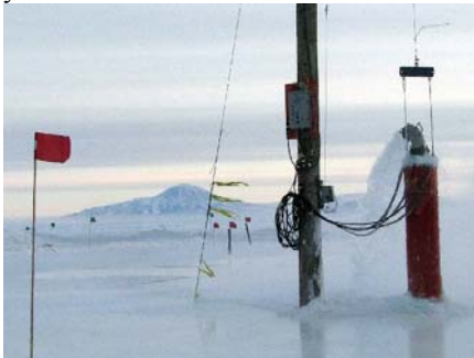
Ice Pier Construction During WINFLY
