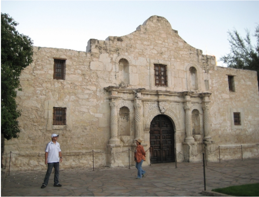
Photo by Dave Hazard
