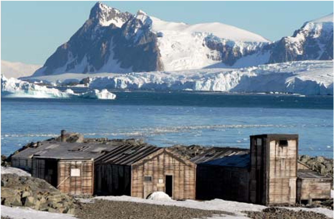
Three surviving buildings of East Base stand abandoned on Stonington Island off the Antarctic Coast.
