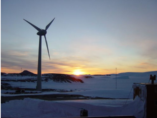
Mawson Station Wind Turbine. Here Comes The Sun
