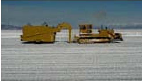
A D-8 tractor tows a 100-ton roller, compacting the snow on Pegasus runway. Photo by Gary Cardullo/Special to The Antarctic Sun
