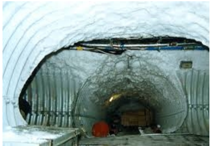
Hallways Inside SANAE III
