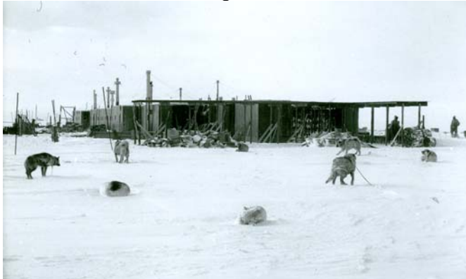
SANAE I under construction
