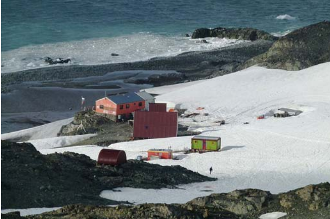
The Bulgarian base in 2012, with the new St. Ivan Rilski Chapel in the foreground and Russian Hut, Lame Dog Hut (light green painted), the Laboratory, Casa España and the Main Building in the background
