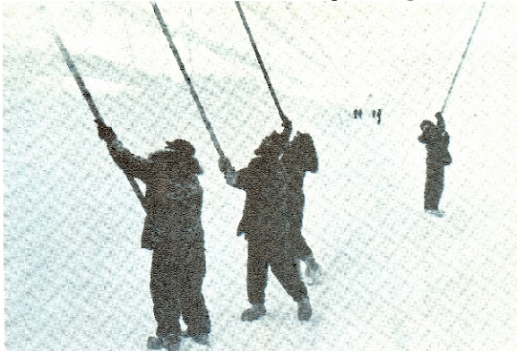
Seabees scraping loose snow from tunnel walls to keep them smooth
